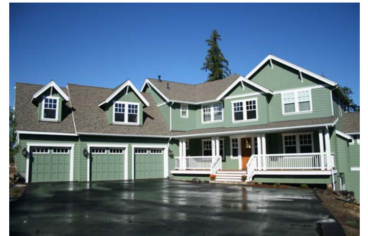
Latest Courtyard custom home—2421 E Grandview Drive—Cd'A 6 bed/6.5 bath/6500 sq ft/movie theater/hi-tech wiring/old-time wood work "It's just like in the magazines..."
